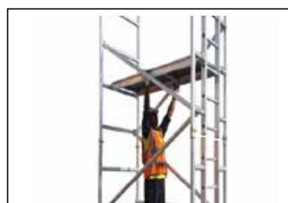
**Step 11** Remove trapdoor platform 1st rung and fit 3<sup>rd</sup> rung from the top and make sure trapdoor opens on the side of ladder frame, apply wind lock system onto the frame rung. (as illustration 3 )
