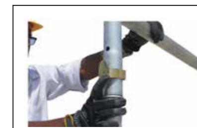
**Step 9** After adding frames engage interlock clips.
