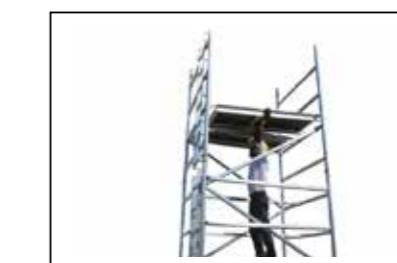
**Step 15** Position platforms at final height of the structure on 3<sup>rd</sup> rung from the top. ensure wind lock systems are in the correct locked position.
