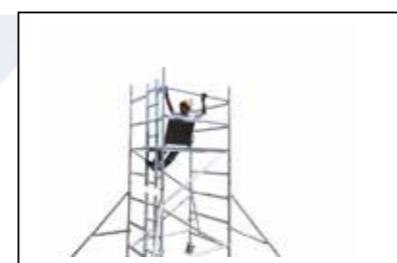
**Step 13** sitting through the door opening of the platforms, position horizontal brace on 6<sup>th</sup> & 7<sup>th</sup> rung On both the open sides of platform. Two on the outer side and two on the mid rungs of the frame.
