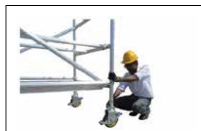
**Step 7** Level the mobile tower, using spirit level. Use adjustable leg of wheel to level the tower.
