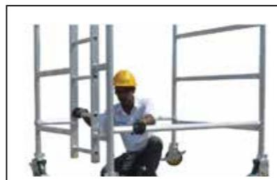
**Step 3** Add two horizontal braces, **BLUE** colour coded to the vertical, member of the frame as low as possible. Both Brace hook line must face from inside towards outside.
