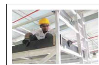
**Step 17** Fit the toe board. Slide the side board into the correct slot in the board. Ensuring the object shouldn't fall and trap door opens fully.
