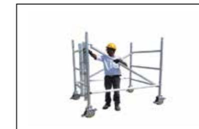
**Step 4** Position two diagonal braces **YELLOW** colour code from first to third rung of each frame in the opposite direction as illustrated.
