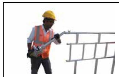
**Step 2** Insert castor and adjustable leg in to the 3 rung span and ladder (or base frame)
