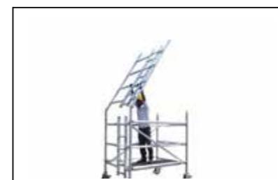
**Step 8** Standing on the platform fit one Span & one Ladder frame, ensuring the ladder frames are in line.
