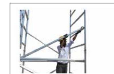
**Step 10** Continue with diagonal brace in zig-zag pattern from 3<sup>rd</sup> to 5<sup>th</sup> and 5<sup>th</sup> to 7<sup>th</sup> rung both the sides in Opposite direction
