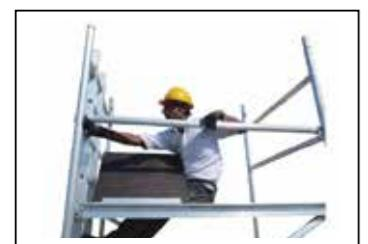
**Step 16** Sitting through trapdoor fit two horizontals on both open sides of the platforms.
