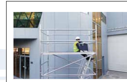
STEP-9 Sitting on the trapdoor opening of the platform fit two horizontal brace on both the open sides of the platform.
