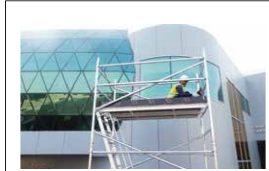
STEP-12 On the final working platform Fit the toe board. Slide the side board into the correct slot in the board. Ensuring the object shouldn't fall and trap door opens fully
