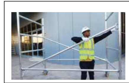
STEP-3 Fit diagonal brace from 1st rung to 3rd on the sides in opposite direction. Make sure braces are aligned. Adjust the wheel nut if necessary to level the tower.
