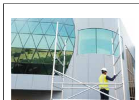
STEP-11 Standing on the guarded platform fit extension frames and follow step 5,6,7,8 and 9 till the desired height in achieved.
