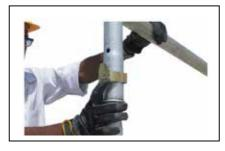
**Step 5**Engage Snap pins to the frames
