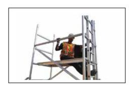
**Step 10** Sitting through the trapdoor add two horizontal braces on 5<sup>th</sup> & 6<sup>th</sup> rung ,two each on both end of the frame.
