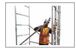
**Step 6** Position diagonal braces YELLOW colour coded From the first rung of both frame in a zig zag pattern from 1<sup>st</sup> to 3<sup>rd</sup> rung & 3<sup>rd</sup> to 5<sup>th</sup> rung either side of the tower opposing each other as illustrated Make sure diagonal brace is aligned.
