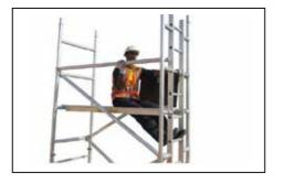
Step 12 Position platform at final height 3rd rung from the top.
