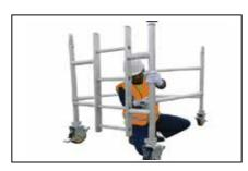
Step 3 Add two horizontal braces, BLUE colour coded, to the vertical member of the frame, as low as possible. All horizontal Brace must fit from inside the tower facing out.
