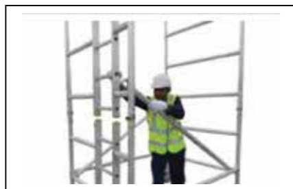
Step 7 Fit two diagonal braces yellow colour coded from 1st rung to 3rd rung of the frame , braces must be positioned in the opposite Direction as shown.
