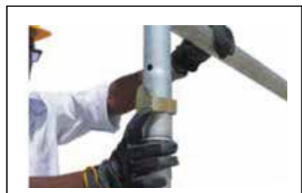
Step 6 After adding frames engage Interlocking clips.
