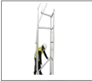
STEP-2 Fit diagonal to connect Podium Frame.
